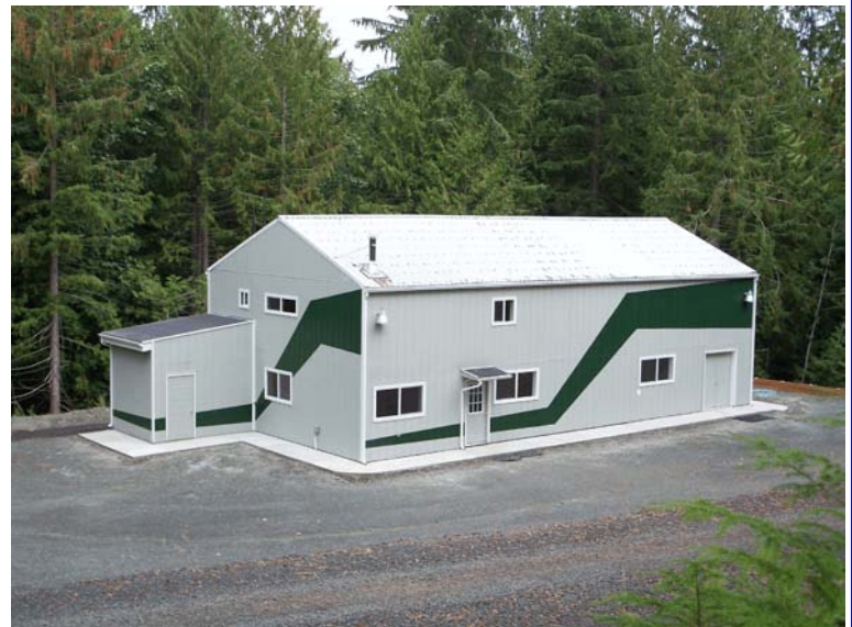
1337 – "Home Enterprise" Facility
